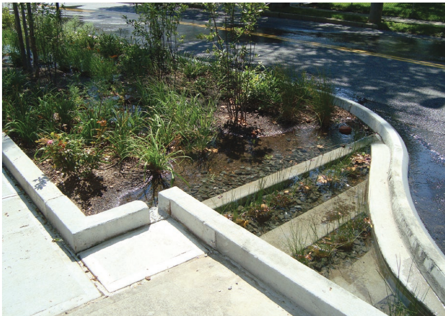
Water can be collected in a forebay, such as the triangular area shown on the right. This allows sediment and debris to settle before the water continues to the planting area: Westbourne Avenue at Bay 25th Street, Queens (Credit: DPR)
