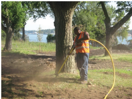
RIGHT: Removing soil from around a tree's roots through pneumatic excavation allows for work to be done without damaging the tree: LEFT - Fort Totten Park, Queens (Credit: DPR); RIGHT - 235th Street and 119th Avenue, Queens (Credit: Lisa Montana)
