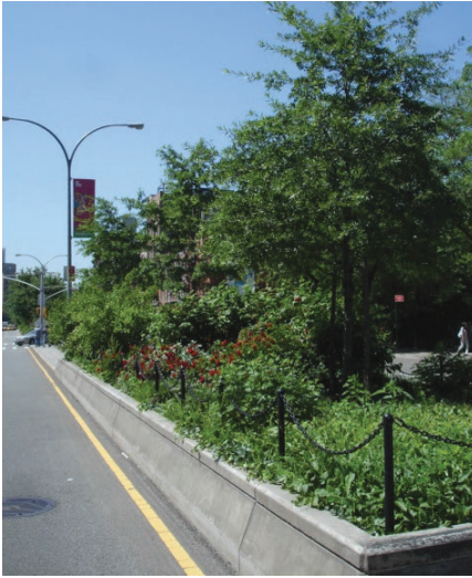
Raising medians to over 12 inches helps accommodate tree roots: West Houston Street, Manhattan (Credit: DPR)
