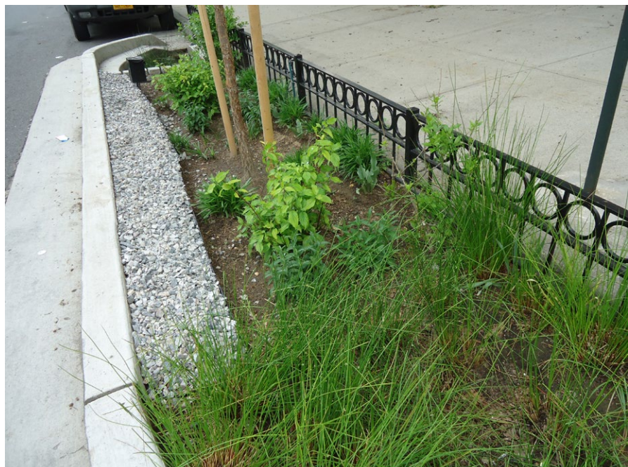
DEP ROW Stormwater Greenstreet constructed in the roadway, modifying the street geometry: Powell Street and Belmont Avenue, Brooklyn (Credit: DEP)
