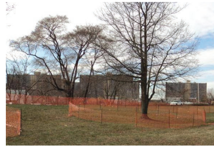
TOP: Tree protection measures during reconstruction of the Allen Street Malls, Manhattan (Credit: DPR)
