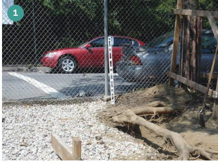
ABOVE: Root pinning resolves sidewalk heaving while preserving existing trees: Black Locust Triangle, 123rd Street and North Conduit Avenue, Brooklyn (Credit: DPR)
