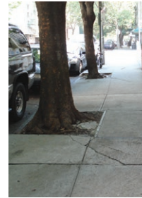
DPR is expanding existing tree beds throughout the city to promote tree health and reduce potential trip hazards created by heaving: Devoe Street, Brooklyn (Credit: DPR)
