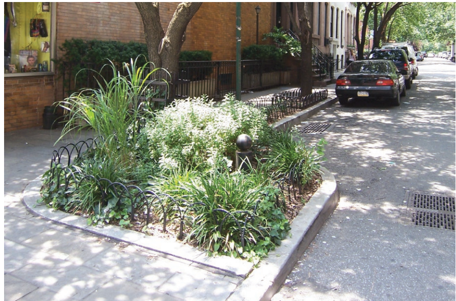
Curb extension with Greenstreet: West 11th Street at Seventh Avenue South, Manhattan
