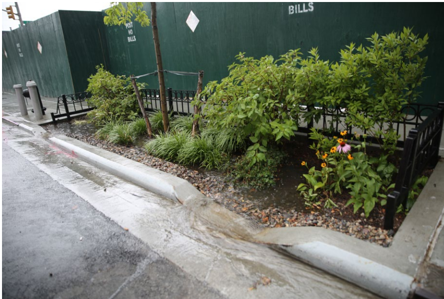
Stormwater entering DEP ROW Bioswale through inlet and overflow exiting from outlet: Dean Street and 4th Avenue, Brooklyn (Credit: DEP)
