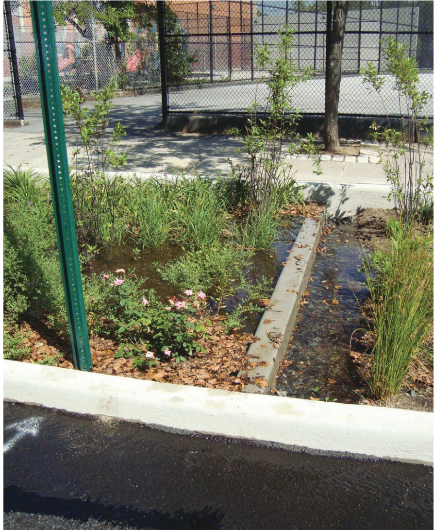
Check dams can separate different levels of a planting area to allow for greater control of slopes and to increase detention: Westbourne Avenue at Bay 25th Street, Queens (Credit: DPR)
