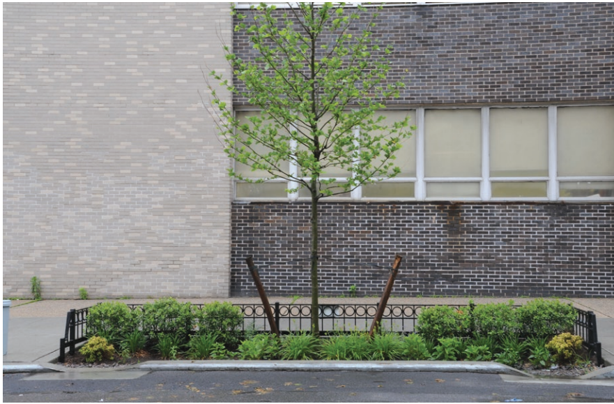
Typical DEP ROW Bioswale with tree: 62nd Drive and Junction Boulevard, Queens (Credit: DEP)
