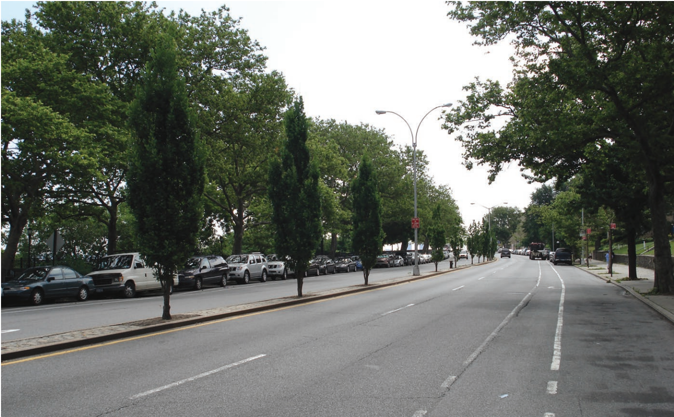
Curb-height median with tree beds. Select narrow species where there is limited space for canopies: Richmond Terrace and Nicholas Street, Staten Island (Credit: DPR)
